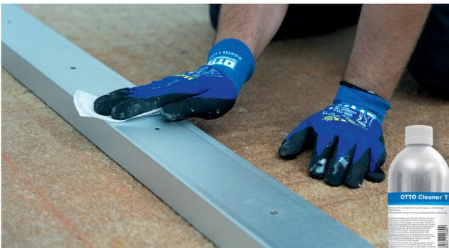
**3 Cleaning the underside of the profile**
