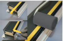
(protective film) from the protruding part and then trim the fixing tape to length. Then leave the liner protruding again and do not completely pull it off.
