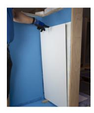
Before attaching the wall cladding panel, the adhesive must first be moistened. This step is not required if a slightly moist, absorbent (but touch-dry) substrate is being used.
