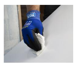
The load-bearing capacity of the substrate is a prerequisite for the bonding of OTTOCOLL® M 595. For absorbent substrates such as cellular concrete, a load-bearing capacity can be achieved by pre-treating with OTTOFLEX Deep Primer. In sanitary areas, direct bonding onto OTTOFLEX Protective Coating is possible. The basic prerequisite for good adhesion is to ensure that the material substrates to be bonded are grease and dust-free, which can be accomplished with a cleaner such as OTTO Cleaner T.
